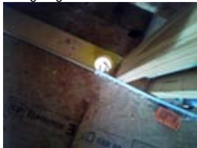
⌋ Missing in concealed spaces every 10 feet horizontal and vertical; blocks not as long, (ex. 2x8 block vs. 2x12 which would match the joists) so not completely blocked in garage horizontal and others marked.
