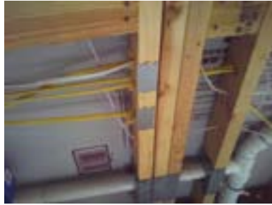
⌋ Missing shoes over notched plumbing pipes which will help bring back to full integrity; missing shoes over drain in living room wall and should be as others;
