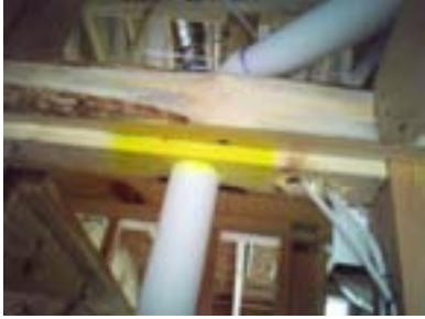
⌋ Missing nail plates over several electrical wires within 1 1/4 inches which were marked and should be like 2nd picture.
