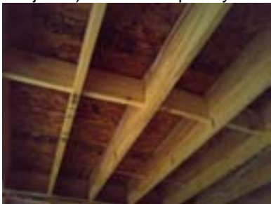
⌋ Missing in concealed spaces every 10 feet horizontal and vertical; blocks not as long, (ex. 2x8 block vs. 2x12 which would match the joists) so not completely blocked in garage horizontal and others marked.
