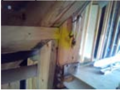
⌋ Missing shoes over notched plumbing pipes which will help bring back to full integrity; missing shoes over drain in living room wall and should be as others;
