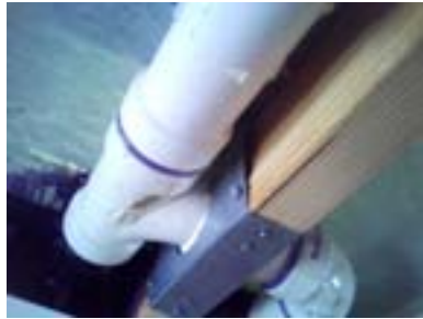
⌋ Missing shoes over notched plumbing pipes which will help bring back to full integrity; missing shoes over drain in living room wall and should be as others;
