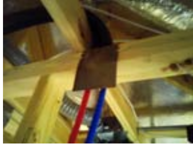
⌋ Missing nail plates over several electrical wires within 1 1/4 inches which were marked and should be like 2nd picture.
