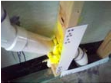
⌋ Missing shoes over notched plumbing pipes which will help bring back to full integrity; missing shoes over drain in living room wall and should be as others;
